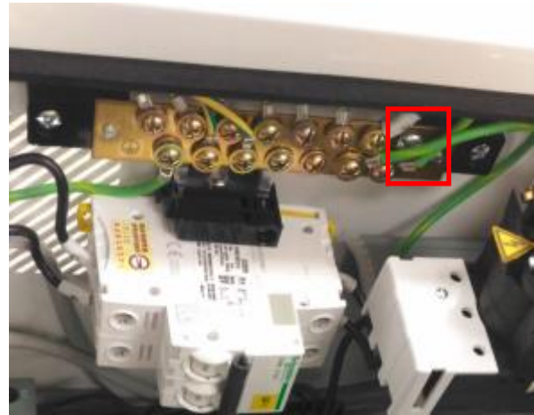
Figure7. 6 Power cable and ground cable installation location
